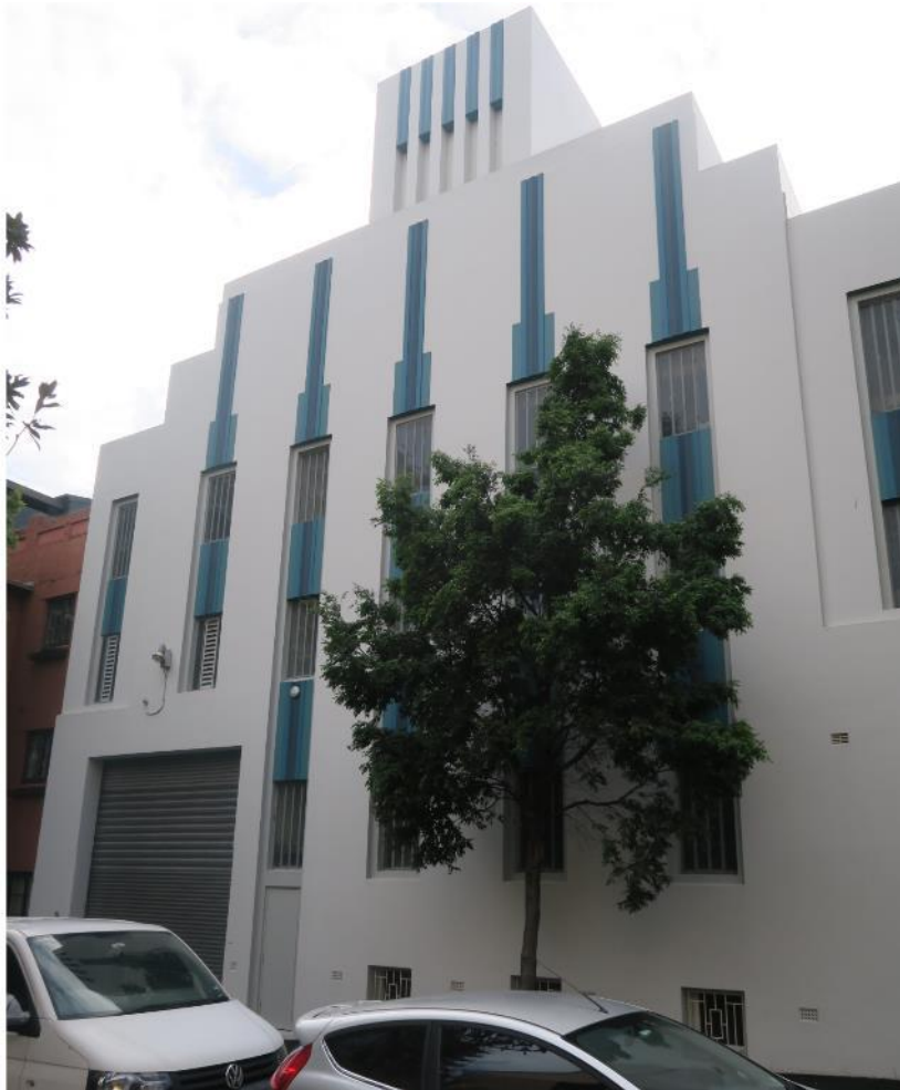
Figure 4: The loading entrance, narrow side stage area, and at the top the access tower to the fly tower (not visible) as viewed from Orwell Street, facing north.
