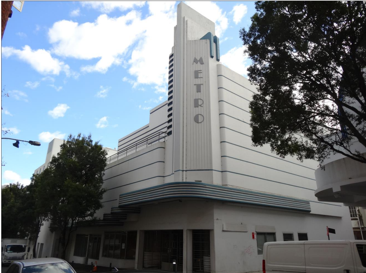
Figure 2: The subject site viewed from the corner of Orwell Street and Orwell Lane, facing north-west.
