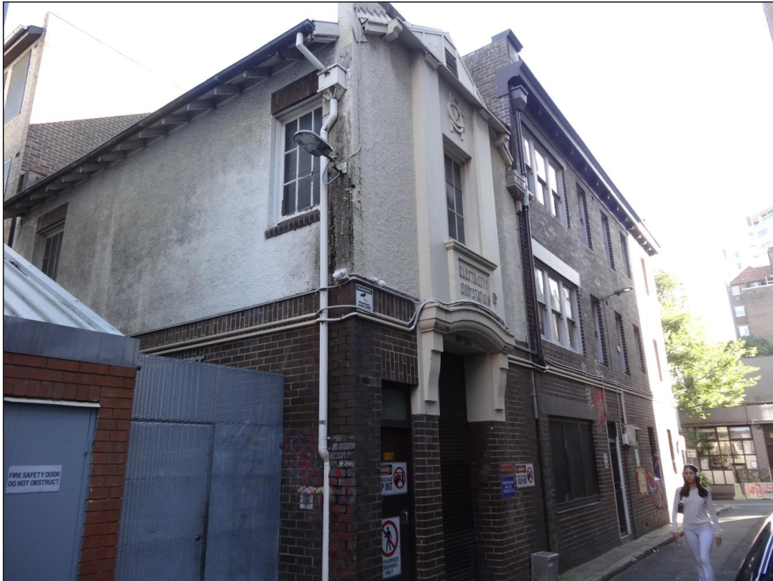
Figure 13: Neighbouring substation and the Wayside Chapel to the north viewed from Orwell Lane.
